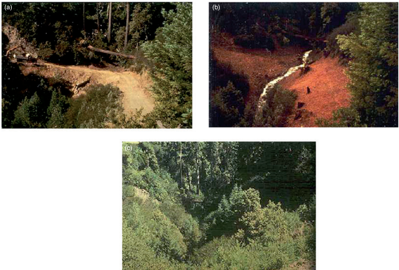
Figure 3. Typical stream channel excavation in the early 1980s. (a) Intact road prism with culvert in place. (b) Following removal of culvert and minor reshaping of streambanks. Minor excavation of stream channel did not reach the original channel bed. No mulch was used. (c) Regrowth of red alder ( Alnus rubra ) 3 years later.
